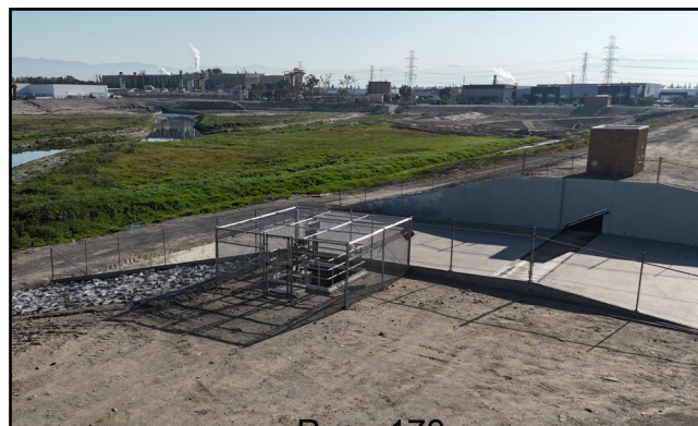
Outlet Control Gate/Rubber Dam System
